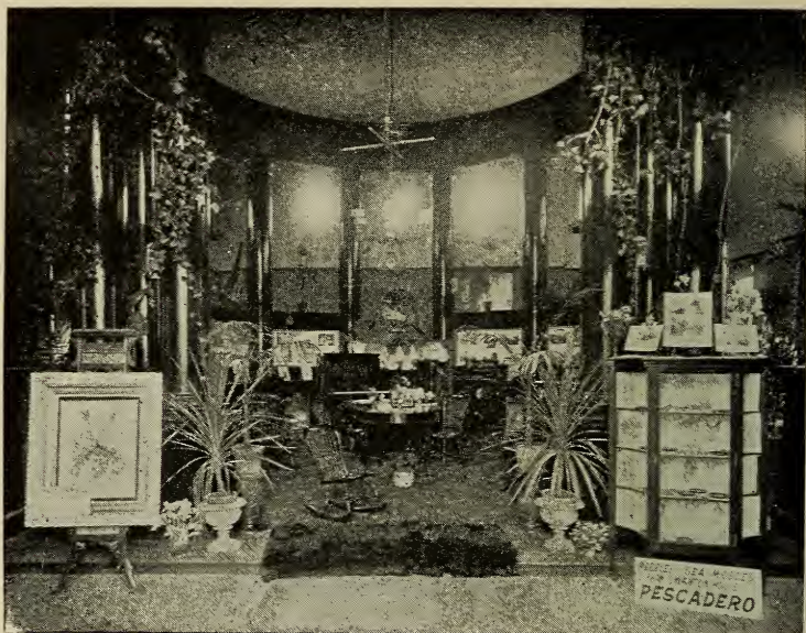
SAN MATEO COUNTY BUILDING—INTERIOR
